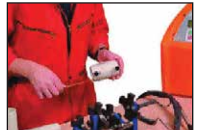
Marking the insertion depth on the pipe
