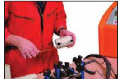
Measuring the fitting insertion depth
