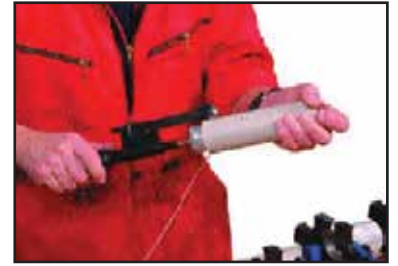
Using the peeling tool to chamfer the pipe
