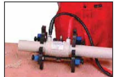
Welding in progress
