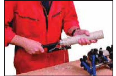
Peeling the pipe end prior to jointing
