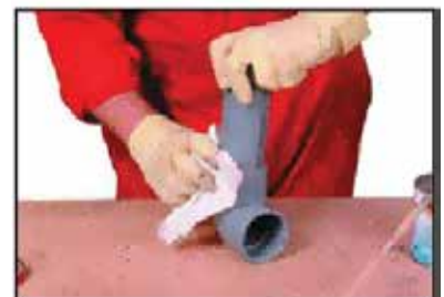
Wiping away excess cement
