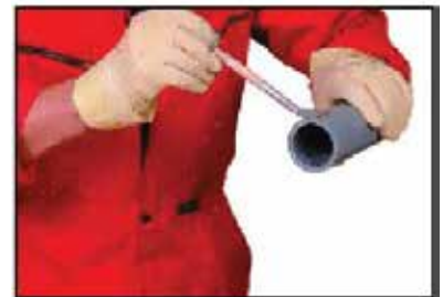
Brush applying cement to the pipe
