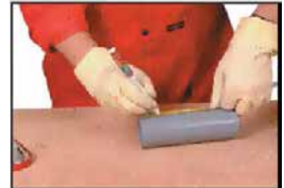
Marking the pipe end
