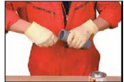
Removing the internal burr
