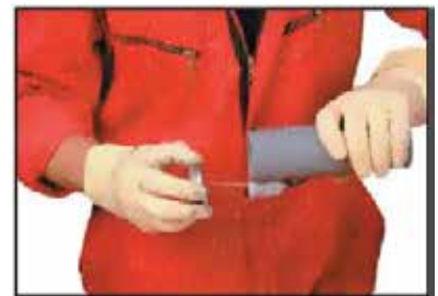
Applying the primer to the pipe
