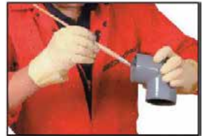
Brush applying cement of the fitting
