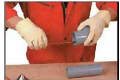
Measuring the insertion depth
