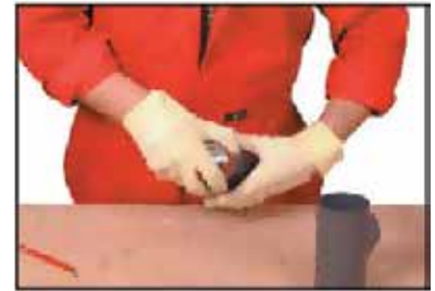
Chamfering the pipe
