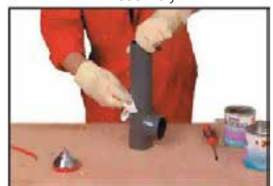
Wiping away excess cement
