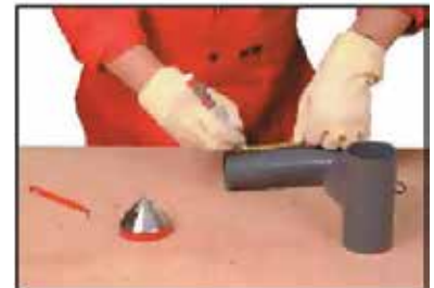
Marking the pipe end
