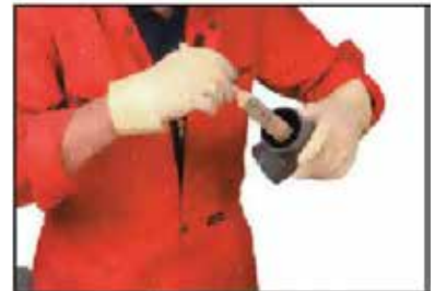
Brush applying cement of the fitting
