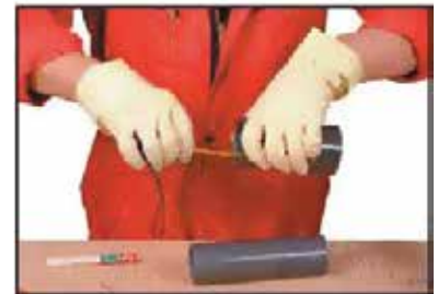
Measuring the insertion depth
