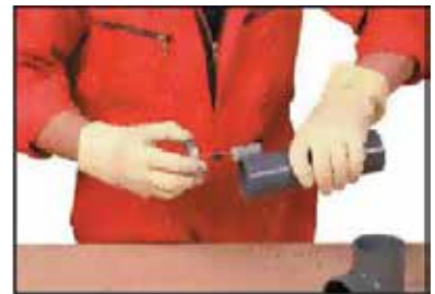
Applying the primer to the pipe
