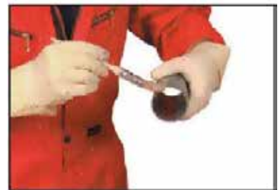
Brush applying cement to the pipe
