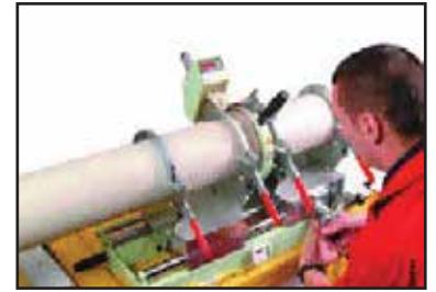
The heating element is brought into place
