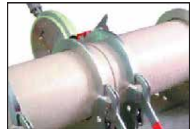
The completed joint is left in the machine during cooling
