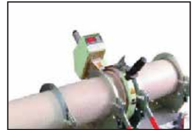
Heating of the pipes
