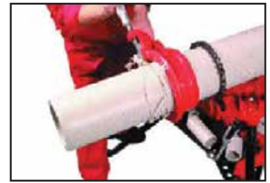
Cutting the pipe with a rotary pipe cutter
