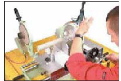
Peeling the pipe
