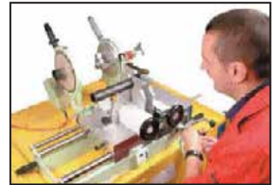
The heater is removed and the parts are brought together
